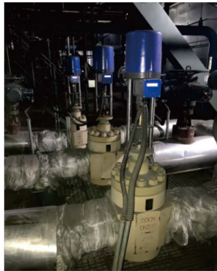
改造后锅炉给水调节阀 Boiler feed water regulating valve after reconstruction
