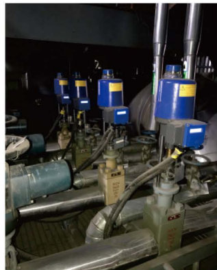
改造后过热器减温水调节阀 Desuperheating water control valve of superheater after reconstruction
